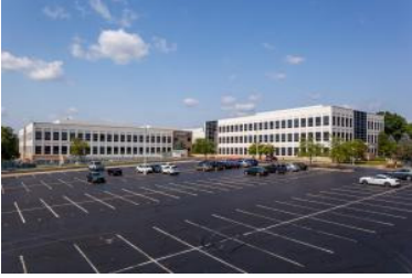
CHASE OPERATIONS CENTER (PHOTO COURTESY OF SENTINEL NET LEASE.)
